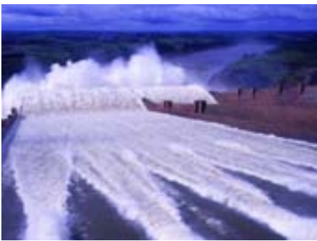
Above Itaipu dam and hydro-electric power station, on the river Parana, Brazil / Paraguay.
