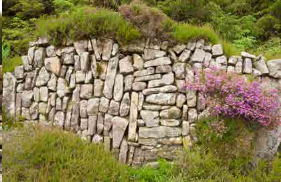
Cláí gaineamhcloiche gan mhoirtéal, Co. Thiobraid Árann. Sandstone drystone wall, County Tipperary.
